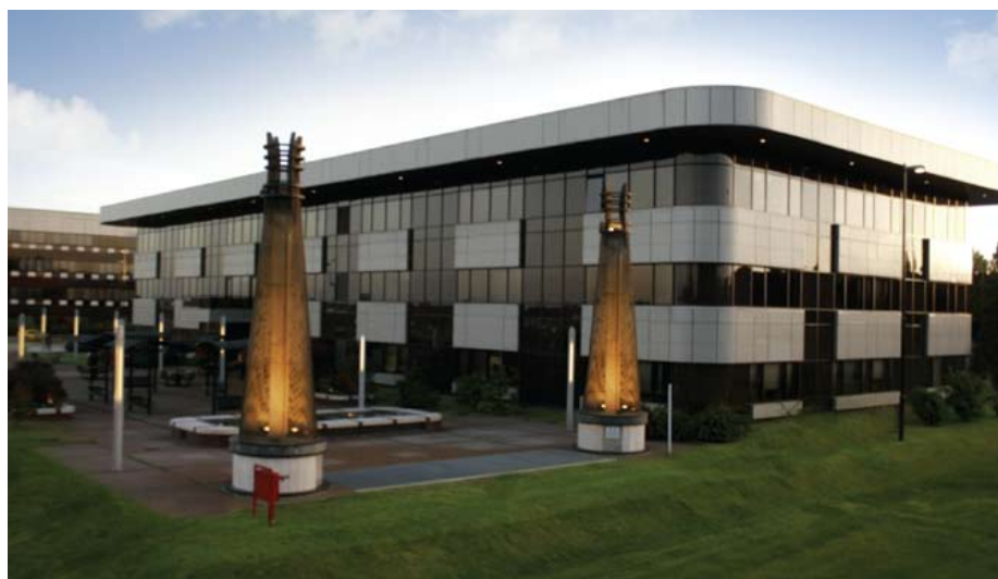
Building @3 (and @1 at the left side of the picture).
